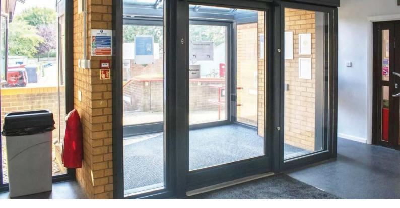
Like all of our communal entrances, we build the frames of our auto-operated doors with high quality stainless steel. We typically fit them with anti-bandit security glazing, which is the appropriate solution for securing most communal entrances.
