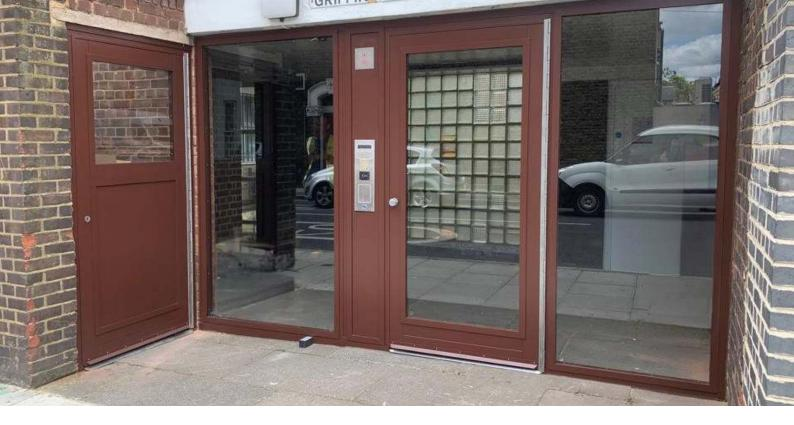
We typically fit our Swing Doors with anti-bandit security glazing, which provides both optimal light and natural surveillance for residents, or the occupants of a building. Securing our Swing Doors with 2 horizontally fitted mag-locks, provides the necessary amount of security for a lower cost. We can also add an optional shear lock.
